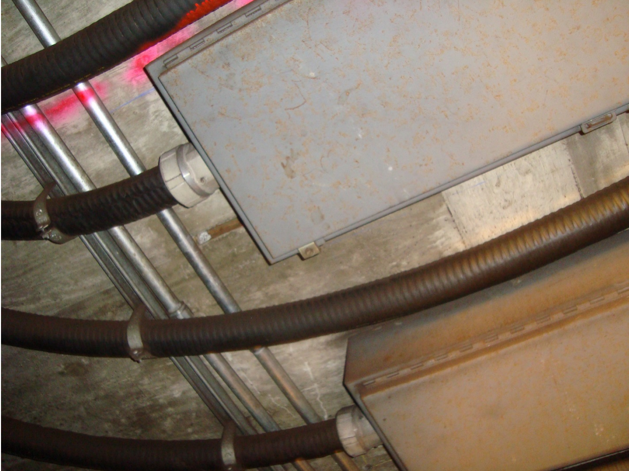
10-Bethesda Plenum, South Elevator pit, looking up, 8-2-2015
