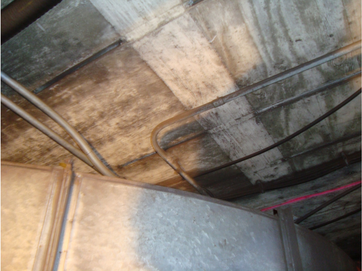
6-Bethesda Plenum, South Elevator pit, looking up, 8-2-2015
