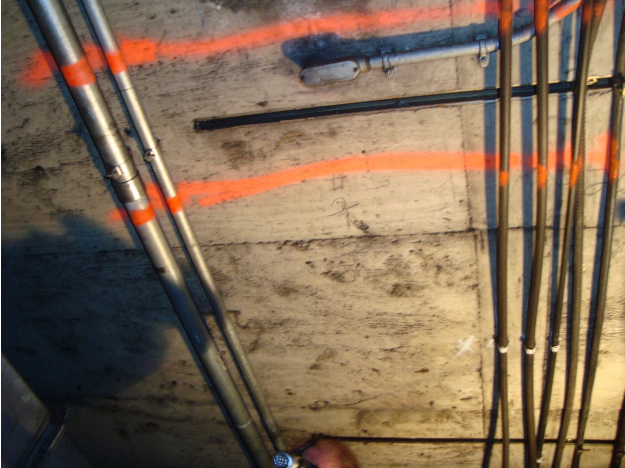
27-Bethesda Plenum, Stair footing, looking up, 8-2-2015
