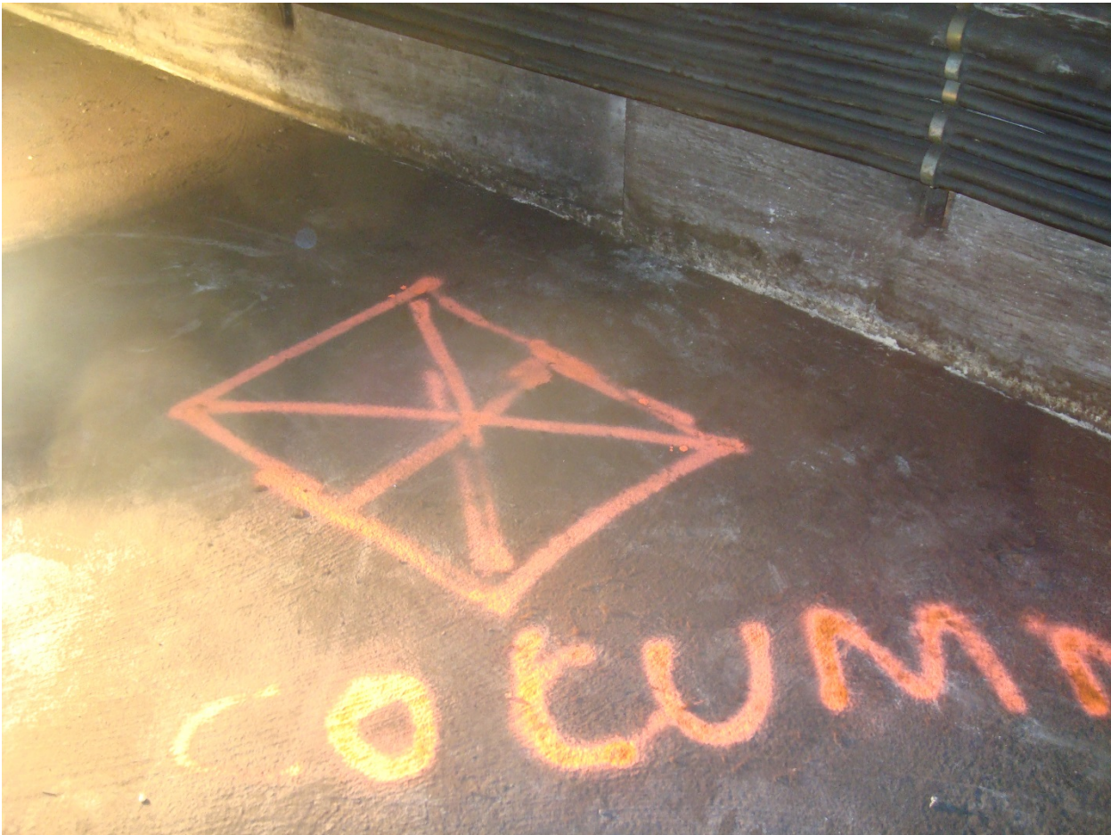
26-Bethesda Plenum, west stair column, looking down, 8-2-2015
