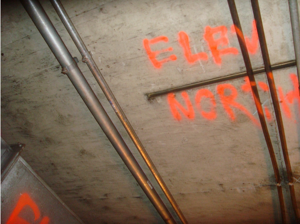
17-Bethesda Plenum, North elevator pit, looking up, 8-2-2015
