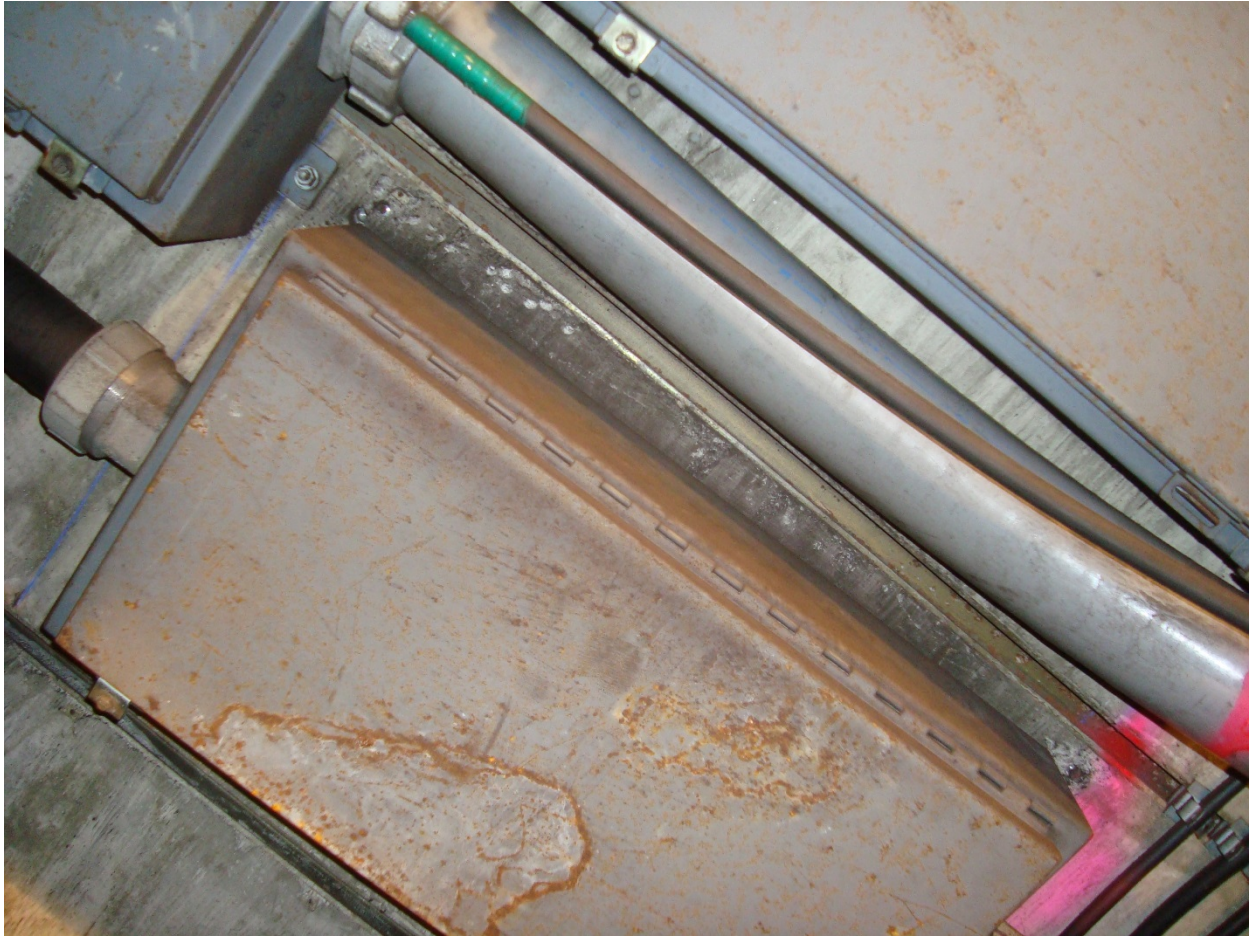
8- Bethesda Plenum, South Elevator pit, looking up, 8-2-2015
