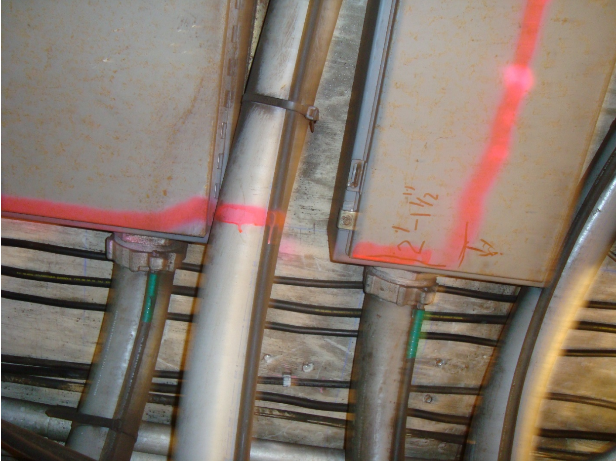
1-Bethesda Plenum, South Elevator pit, looking up, 8-2-2015
