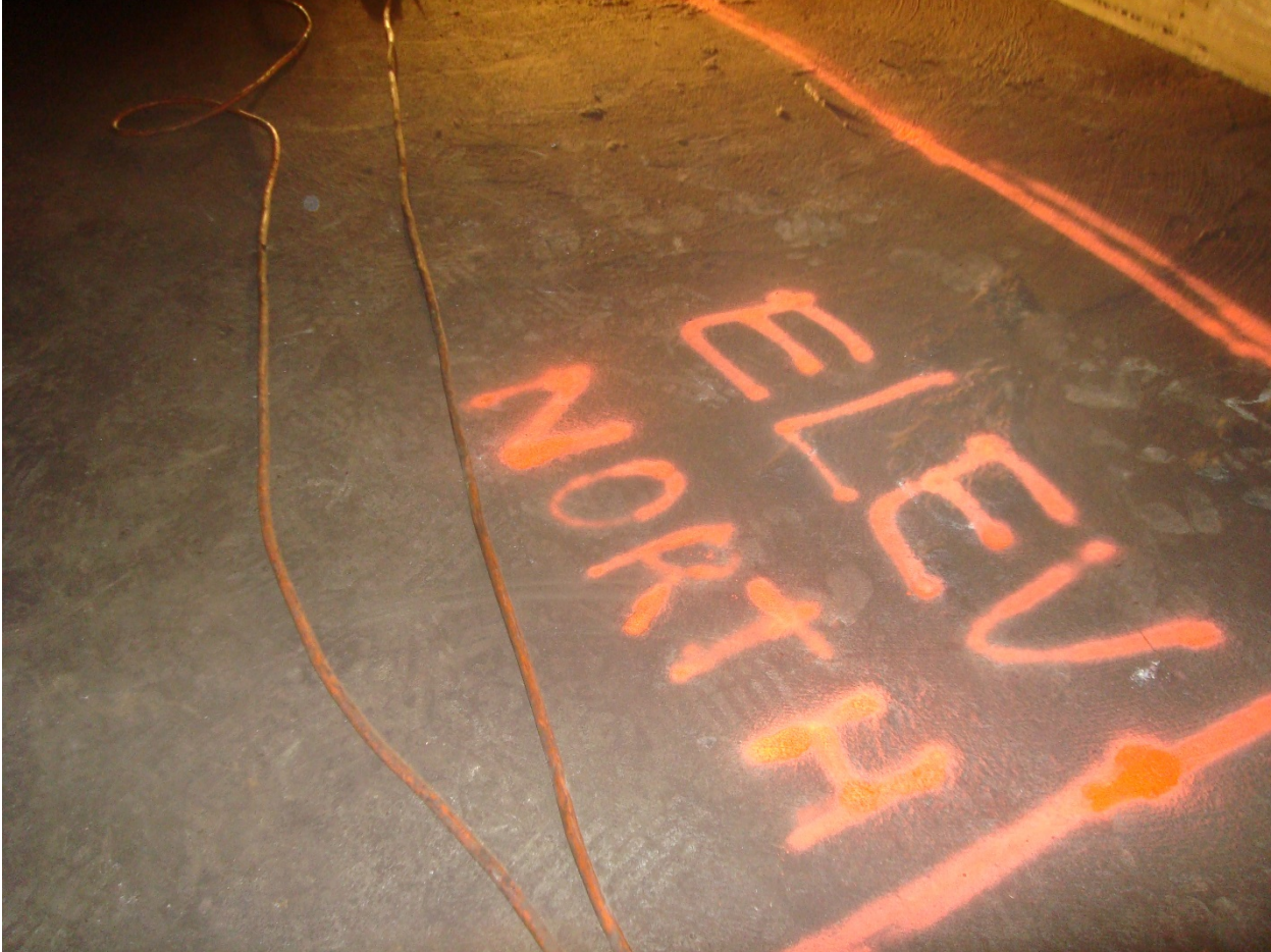
18-Bethesda Plenum, North Elev. Pit, looking down, 8-2-2015
