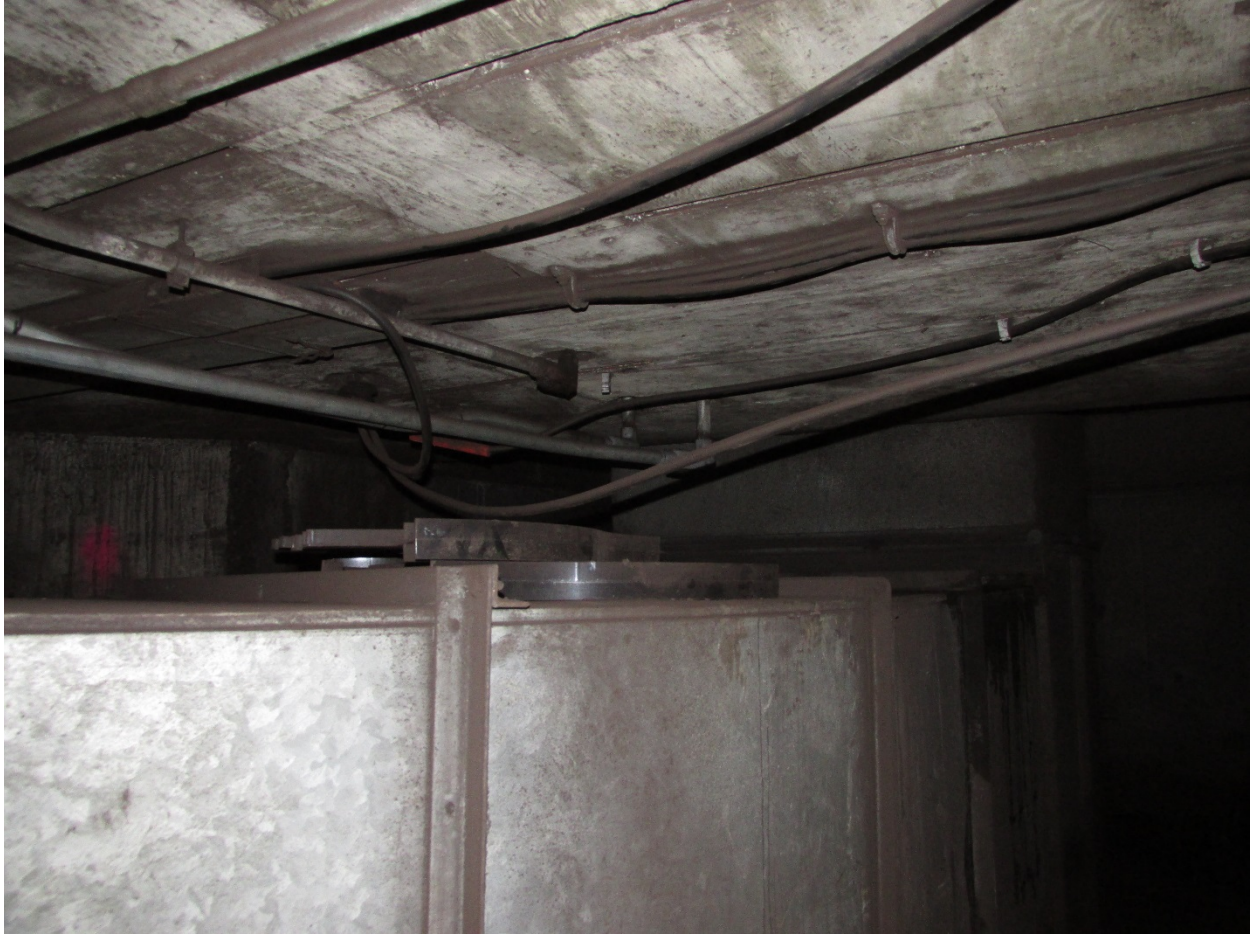
A09 Platform South Side Plenum looking towards South Wall
