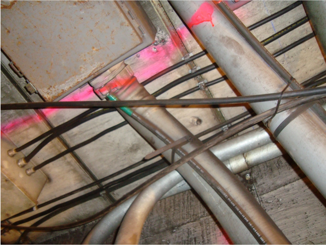
2-Bethesda Plenum, South Elevator pit, looking up, 8-2-2015
