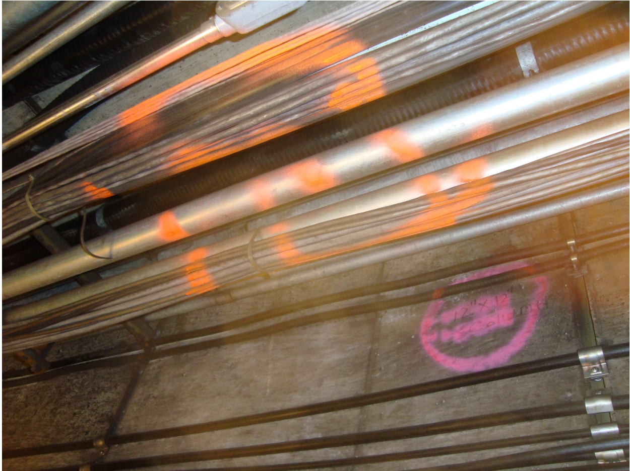
25-Bethesda Plenum, West stair column, looking up, 8-2-2015
