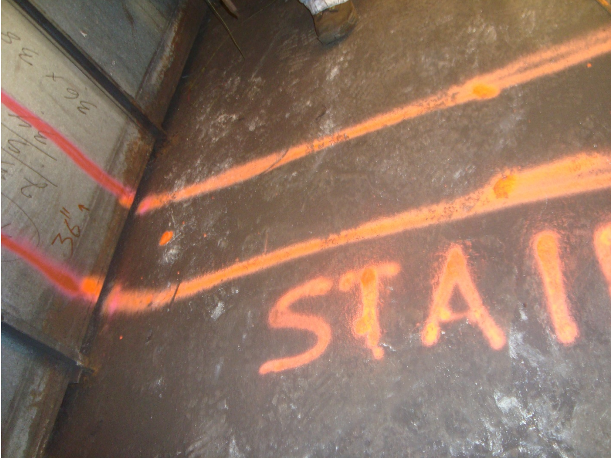
30-Bethesda Plenum, Stair footing , looking down, 8-2-2015
