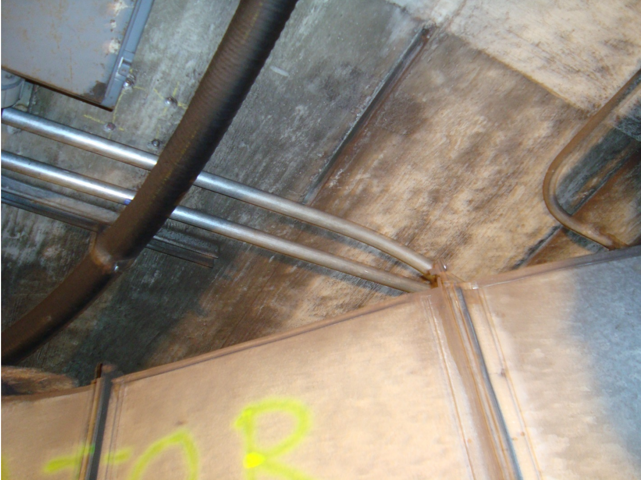
5-Bethesda Plenum, South elevator pit, looking up, 8-2-2015
