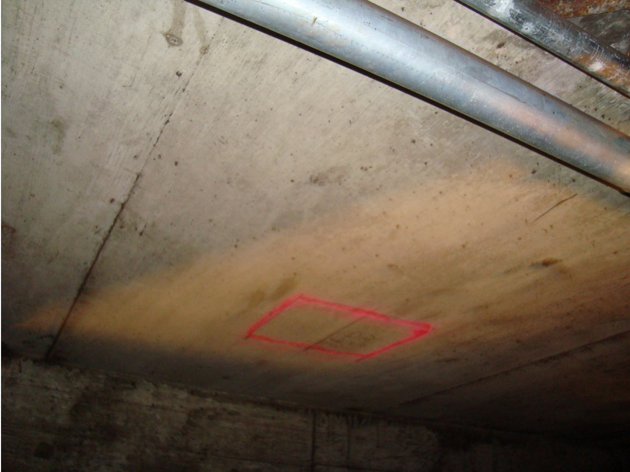
24-Bethesda Plenum, East stair column, looking up, 8-2-2015
