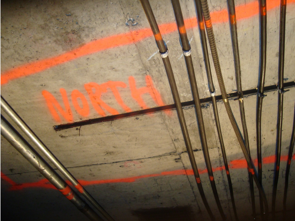
33-Bethesda Plenum 5'X2' Mezz. columns looking up, 8-2-2015
