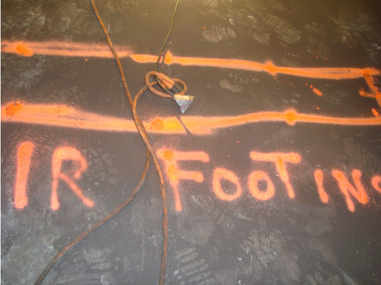
29-Bethesda Plenum, Stair footing, looking down, 8-2-2015
