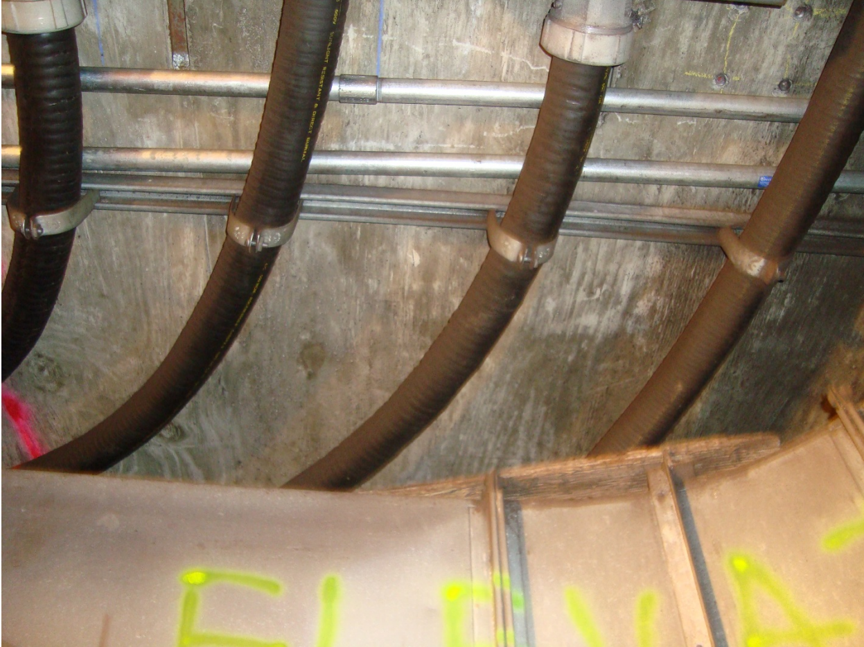
4-Bethesda Plenum, South Elevator pit, looking up, 8-2-2015
