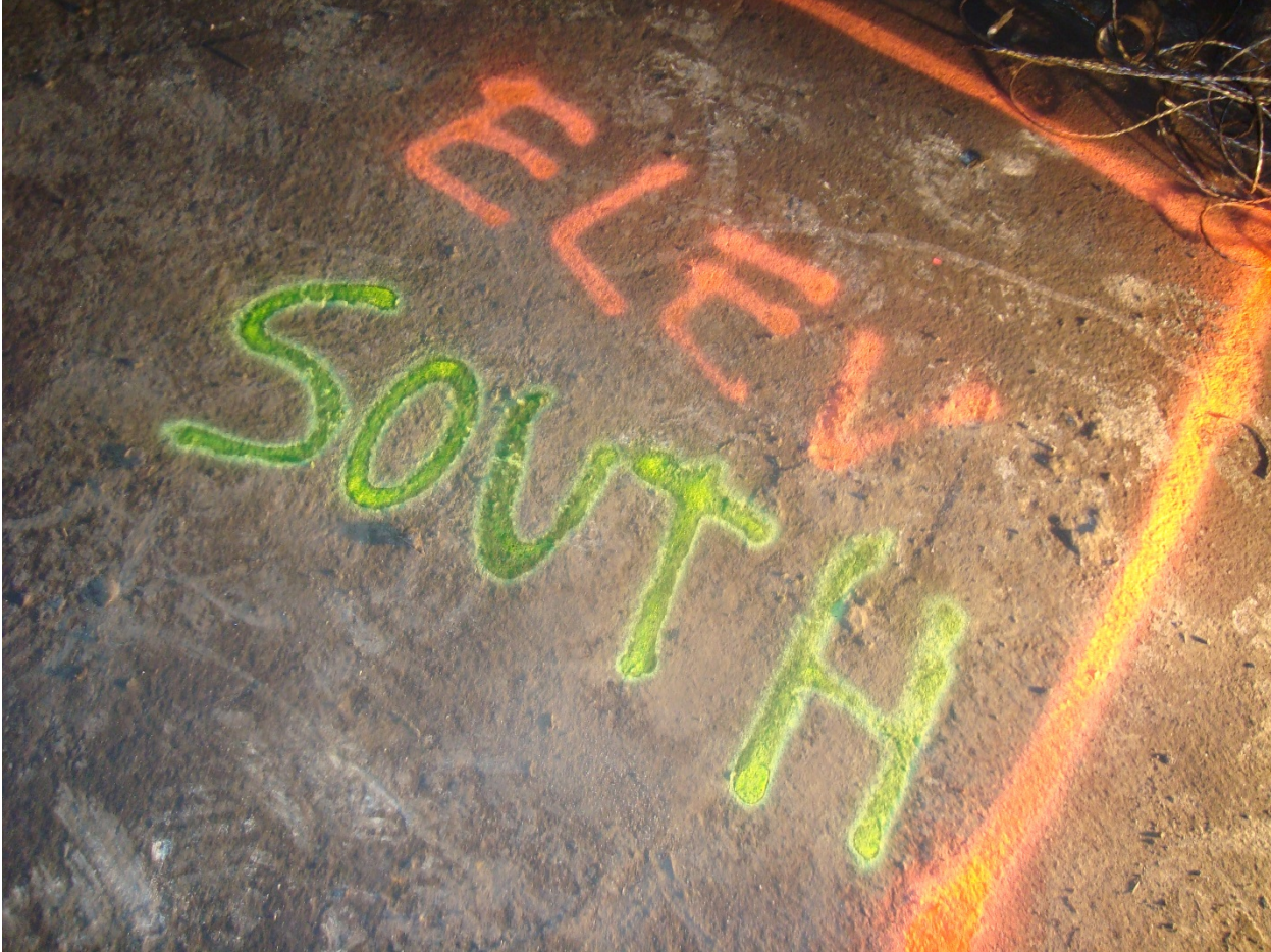
13-Bethesda Plenum, South Elevator pit, looking down, 8-2-2015
