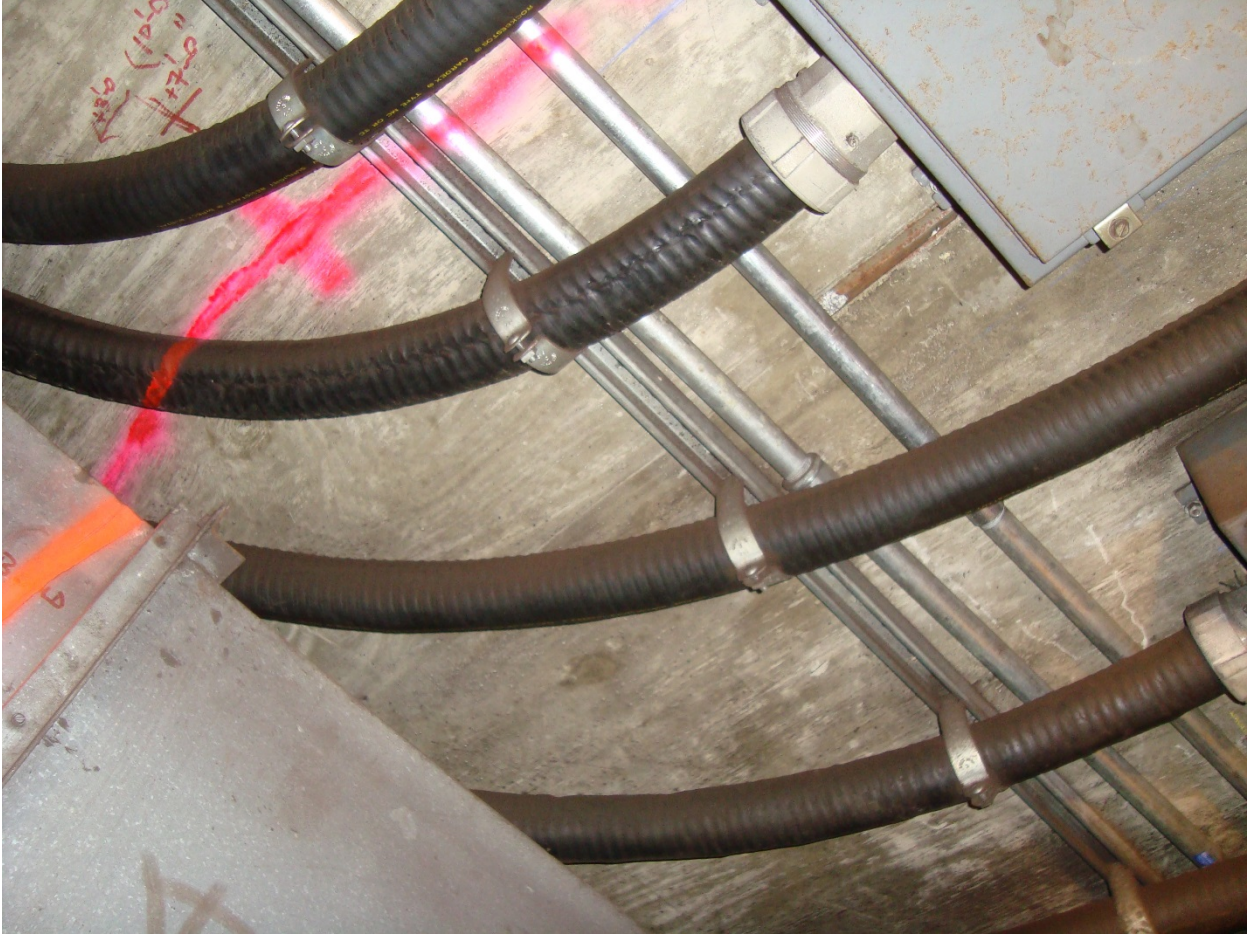
9-Bethesda Plenum, South Elevator pit, looking up, 8-2-2015
