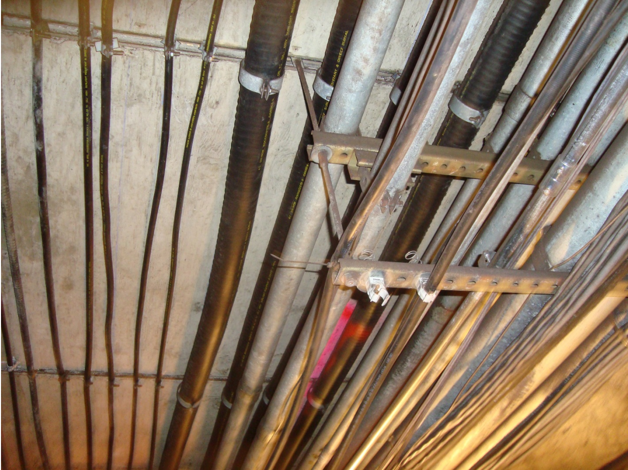
16-Bethesda Plenum, North elevator pit, looking up, 8-2-2015
