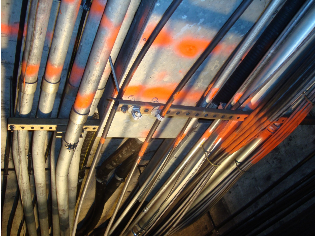
28-Bethesda Plenum, Stair footing, looking up, 8-2-2015
