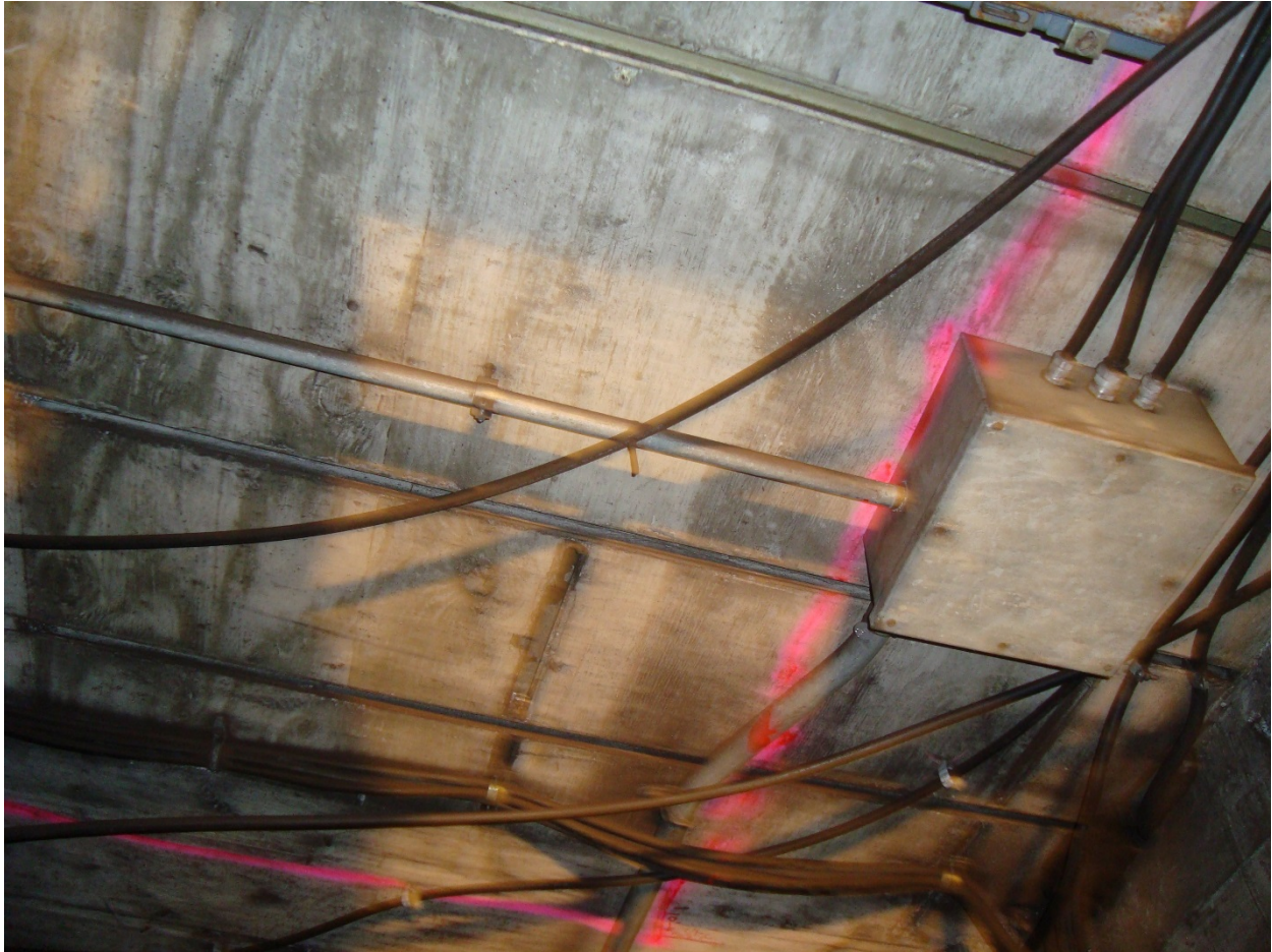
7-Bethesda Plenum, South Elevator pit, looking up, 8-2-2015
