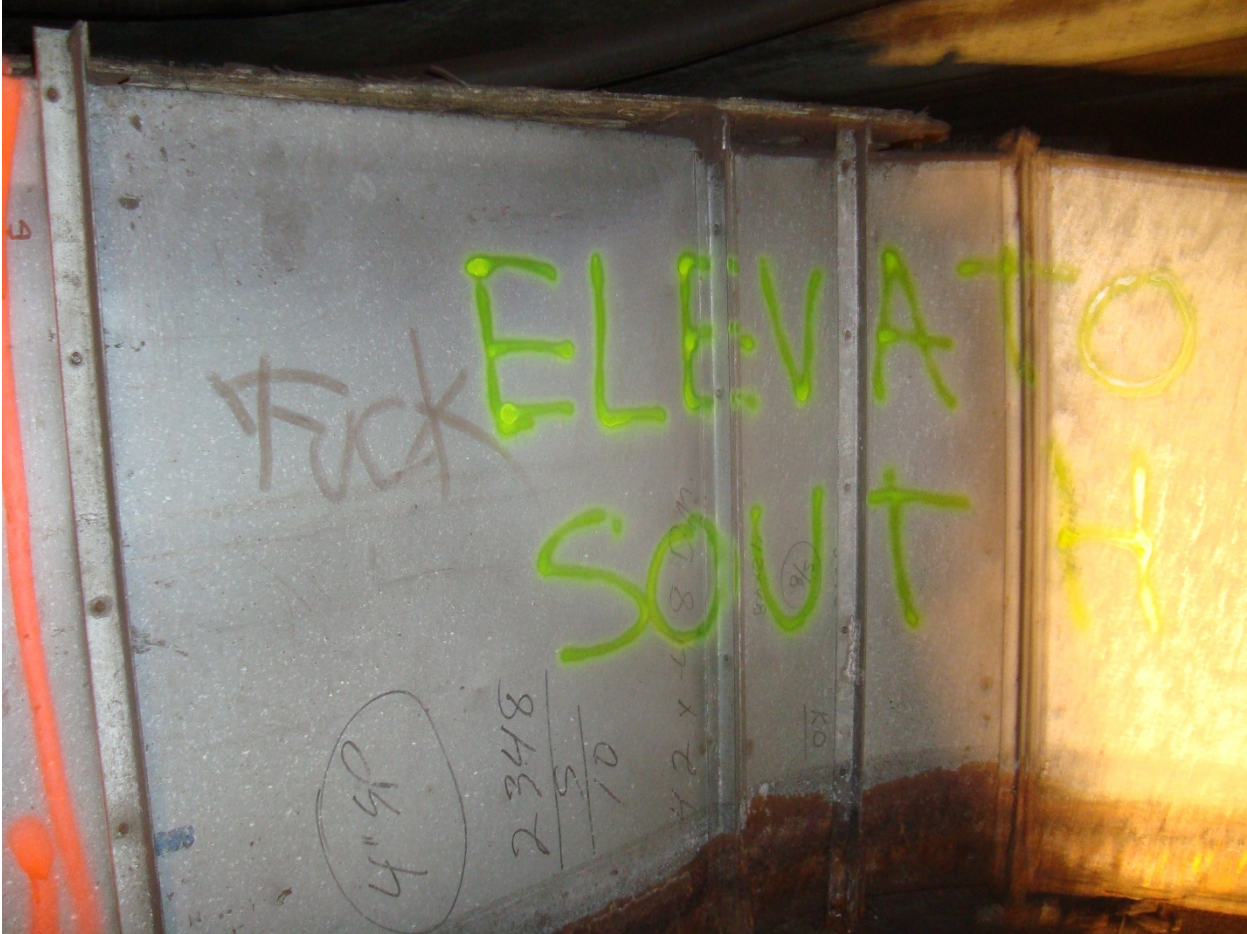
12-Bethesda Plenum, South Elevator pit, looking East, 8-2-2015
