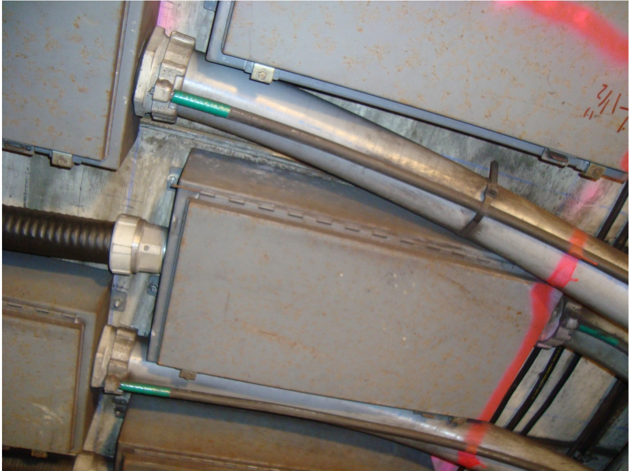
11-Bethesda Plenum, South elevator pit, looking up, 8-2-2015
