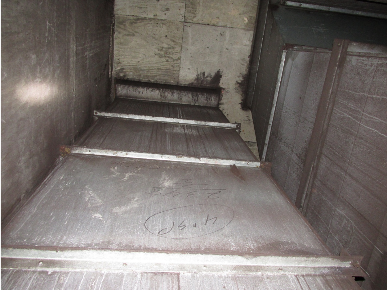
A09 Platform South Side Plenum South End wall shaft looking up
